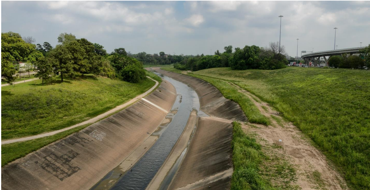
Figure 1: Typical View of White Oak Bayou Downstream from Taylor Street Bridge
